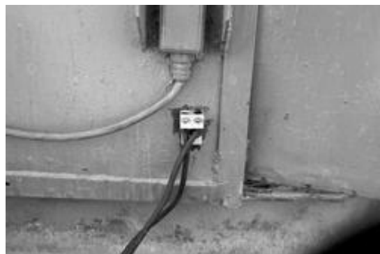
Note: double metal-to-metal connection
