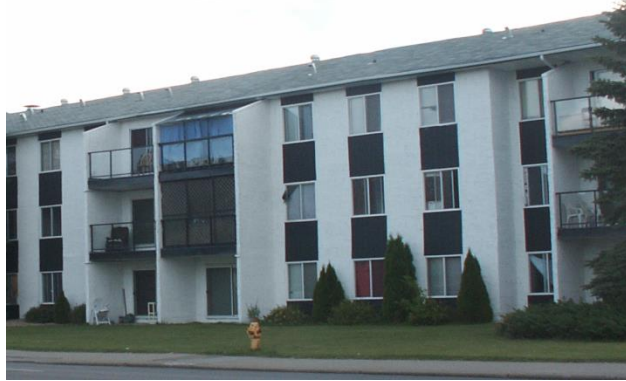
Figure A-1-2-1 Three-storey apartment building
