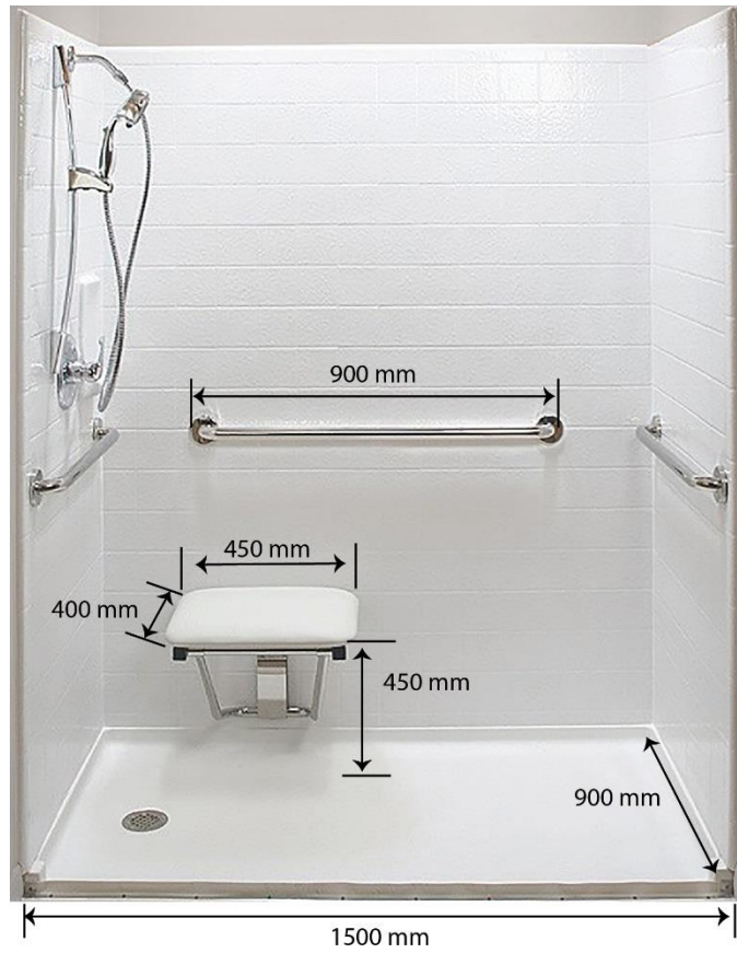
Figure A-7-1-1 Measurements of shower requirements [Sentence 3.8.3.13.(1)]
