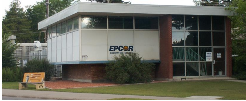
Figure A-1-2-6 Substation
