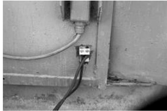
Note double metal-to-metal connection
